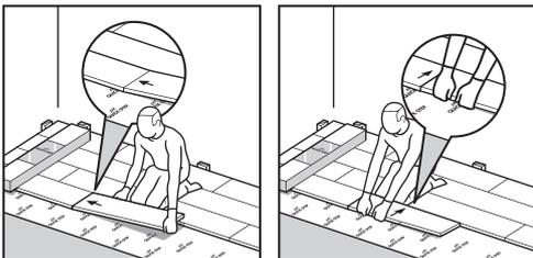
In places where it is too difficult to install the Uniclic® planks with the tapping block (e.g. against the wall), you can tap them together using the pulling iron and a hammer.
